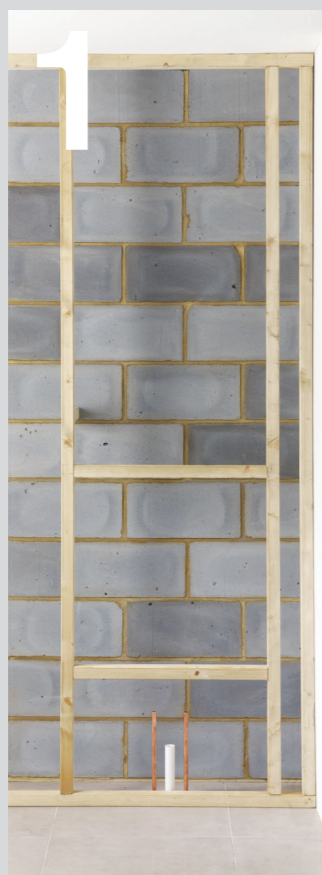
01 Install timber-frame (supplied by others).
