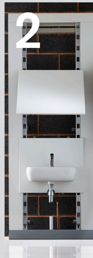
02 Click-fix the first Vepps unit onto the frame and slide into position. Open the mid panel to a fully hinged position. Attach a vertical flashgap to the frame on either side of the unit, screw-fixing to the frame from the face. Fix tie back to the wall. Repeat until all units are in place.
