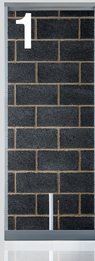
01 Once the site has been prepared, fix the aluminium docking frame to the wall, ceiling and floor.
